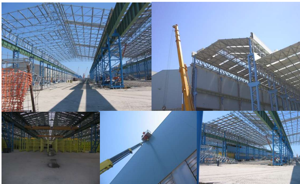
Industrial Company MARCEGAGLIA Ravenna -RA-
