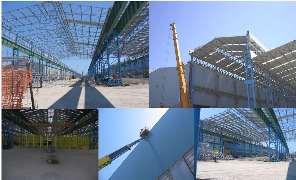
Industrial Company MARCEGAGLIA Ravenna -RA-
